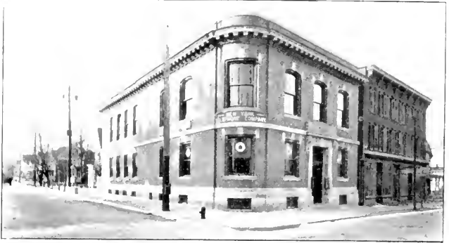
NEW YORK TELEPHONE BUILDING.
